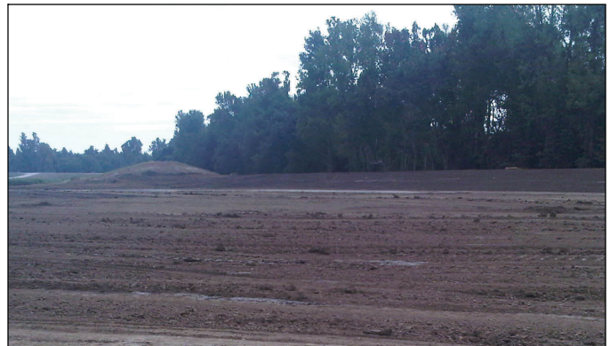
A nearly-complete levee segment at the upper crevasse. Quality-Assurance inspectors will verify that this segment complies with our requirements for interim elevation and cross section.
