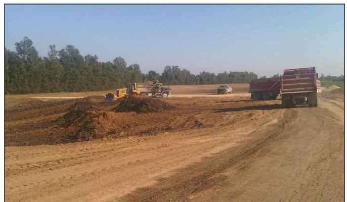
Placing clay into the third of five scour holes Sept. 12. Crews previously filled the hole to the water table with sand, and are now placing clay in the hole to provide a stable base for the levee and to resist seepage.
