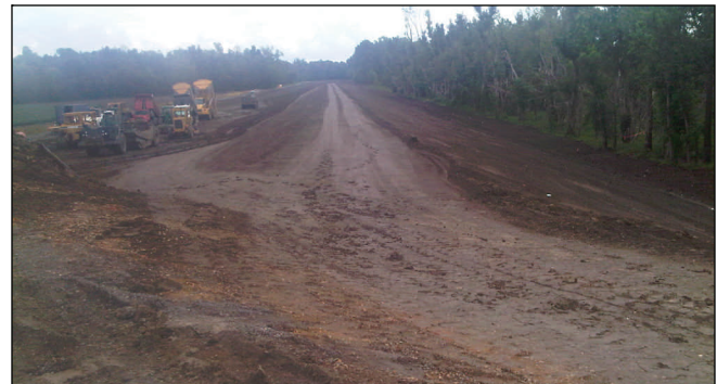
Today was wet and muddy at the lower crevasse. Crews halted earthwork due to the wet conditions, focusing on road and equipment maintenance instead.
