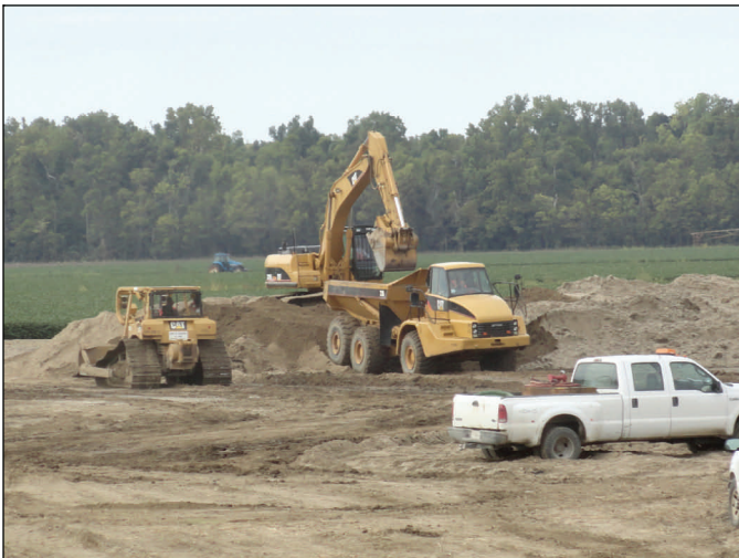
Harvesting sand at the center crevasse Friday. Crews are harvesting sand deposited on the surrounding land during the flood for use as fill material.
